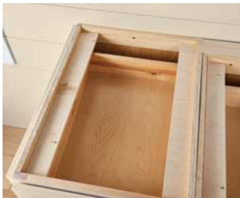
I-beam supports improve base cabinet stability
